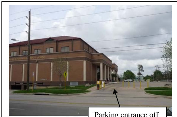
Parking entrance off of Hermann Drive
